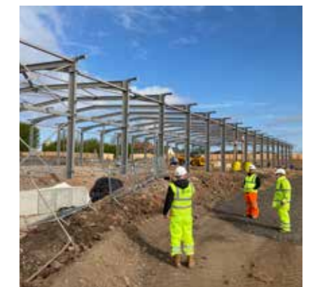
Improvement works, Skelmersdale town centre
