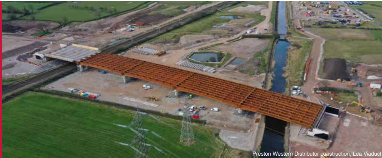
Preston Western Distributor construction, Lea Viaduct
